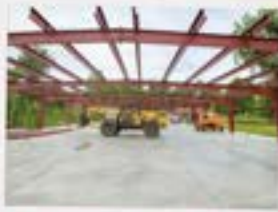
2019 - Construction of new facilities at 531 Belvedere Clearwater Rd began
